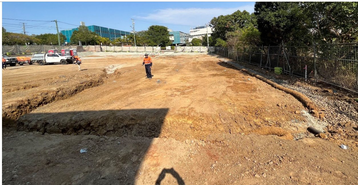
Plate 3: Natural soil materials comprising red/brown silty clays
