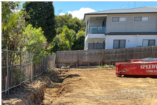
Photograph showing excavated service trench along the northern boundary and the exposed sewer main at the end of the trench. A gravel drain was installed by EPS in the service trench shown (refer to Figure 12, Appendix A).
