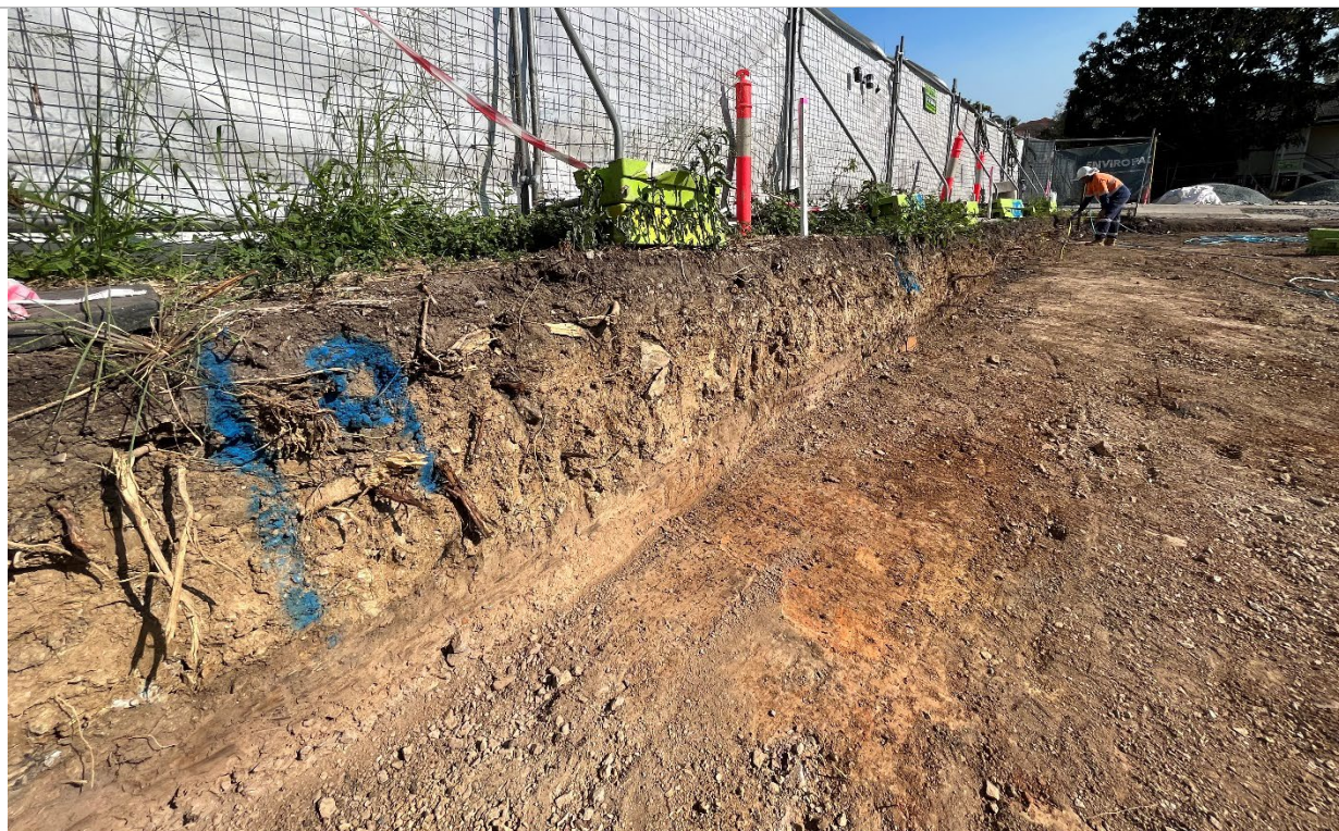
Excavation along the western boundary of the Site. The survey peg shown is offset 0.5 m west off the Site boundary.
