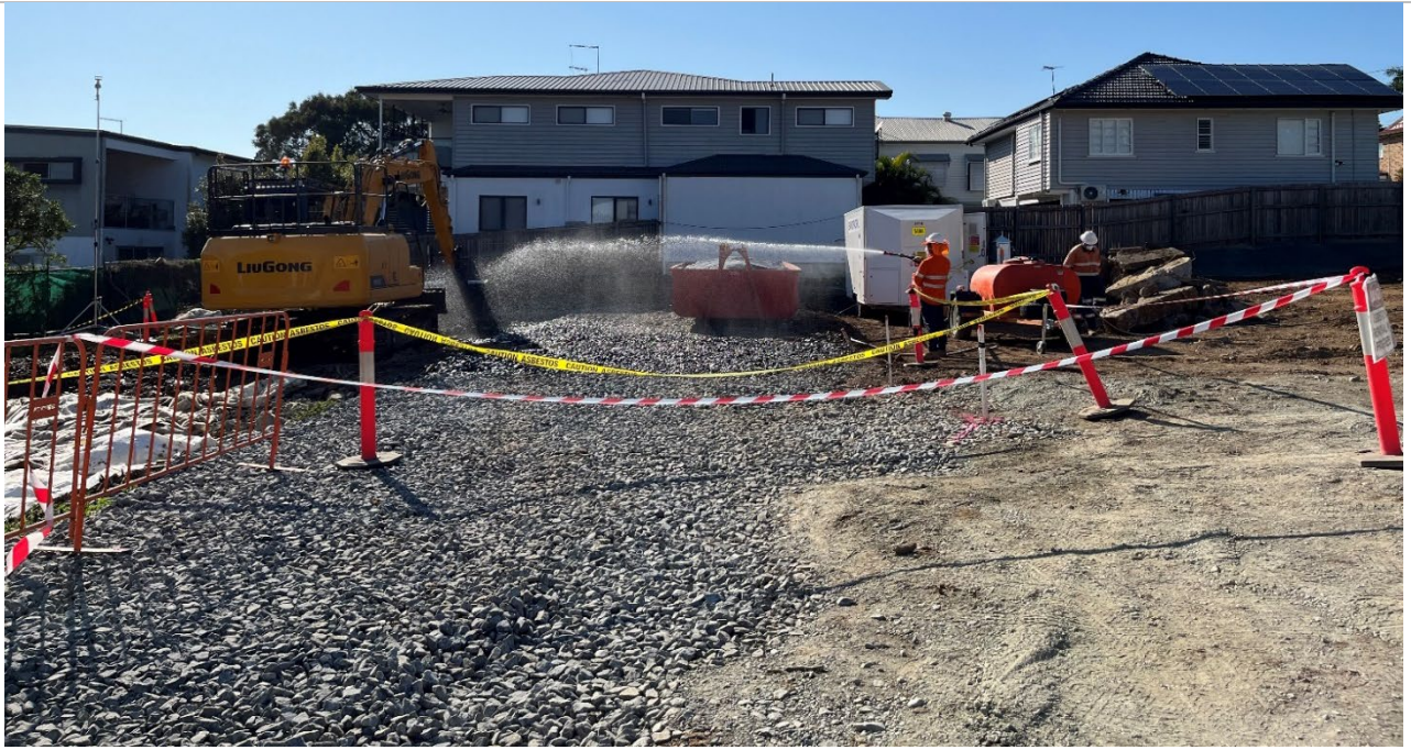
Plate 4: Active dust suppression during site excavation works along the eastern boundary
