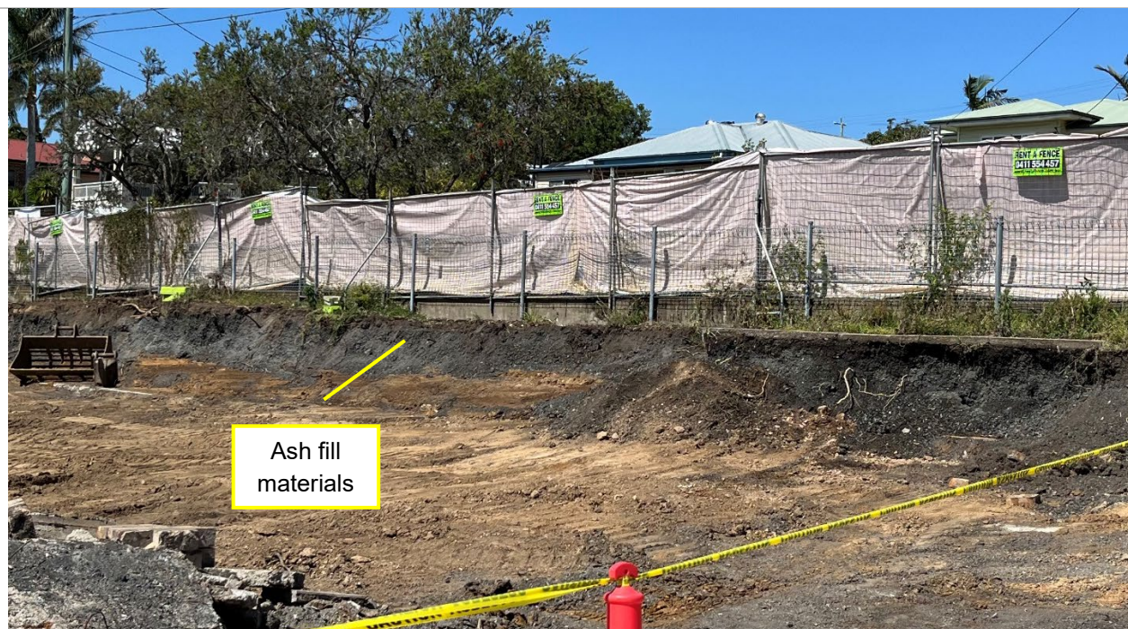
Plate 2: Excavation of ash fill materials during remediation along the southern boundary of the Site during remediation
