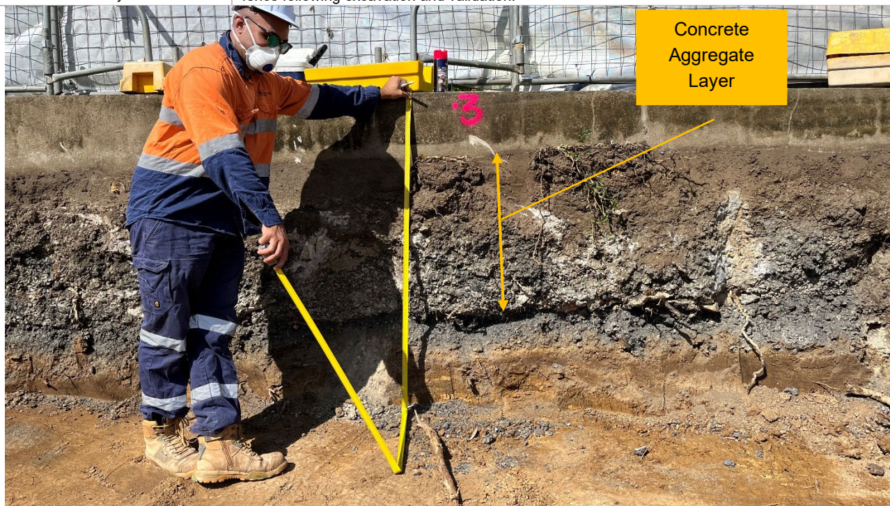
Excavation along the southern boundary was undertaken to the retaining wall which was the practicable limit of excavation.
