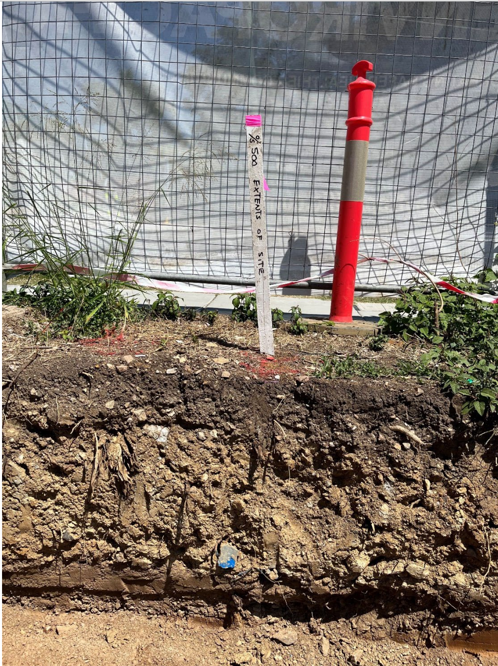
Excavation along the western boundary of the Site. The survey peg shown is offset 0.5 m west off the Site boundary.
